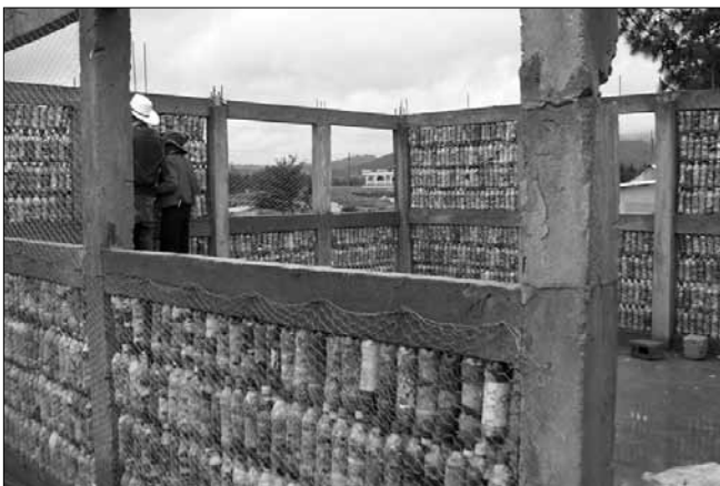
A "bottle school" under construction in Guatemala.
